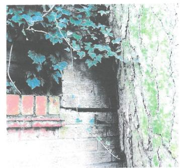
scheme that was proposed by Ward Cole did not address the fact that the trees at the time were in contact with the wall and specifically the parapets that were fractured horizontally by the direct contact of the trees were not reinforced. Therefore, inevitably, further damage has occurred to the wall leaving the parapet, where trees are in contact with the wall. in dangerous enclose condition. 1 photograph of the parapet location and note that the
